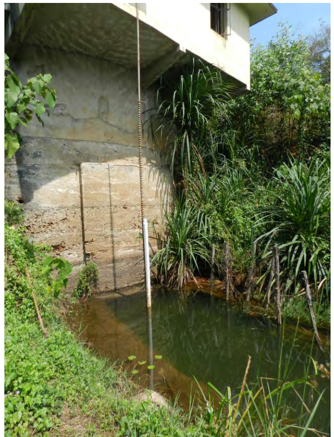
Lake level monitoring station at pump house
