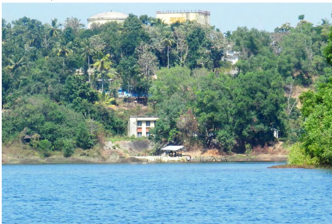
Pumphouse for water supply to Kollam City
